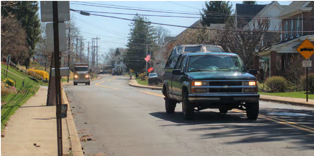
Main Street Existing Conditions
