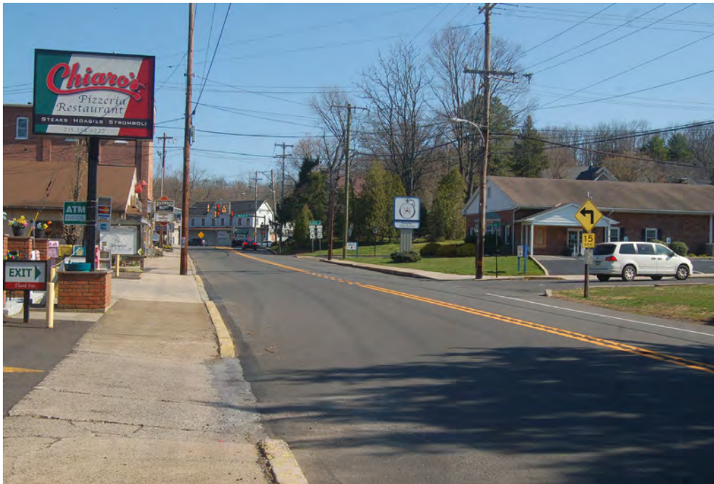
PA 29 Gravel Pike Existing Conditions
